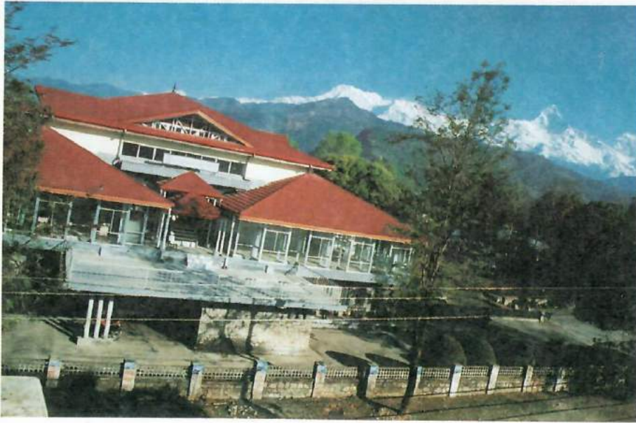
Nepal Rastra Bank Branch Office Building , Pokhara
